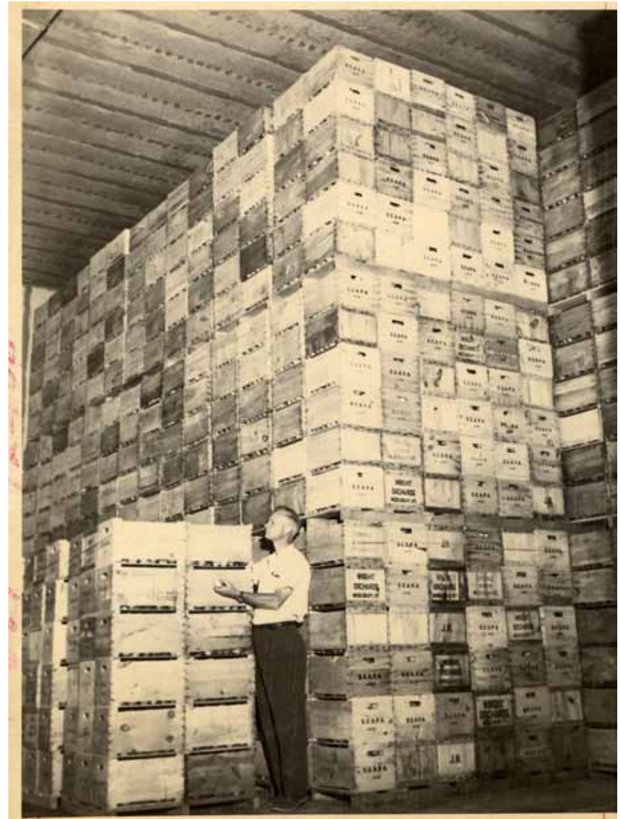
Wright Orchards (Middlebury) apple storage facility (Date unknown).
