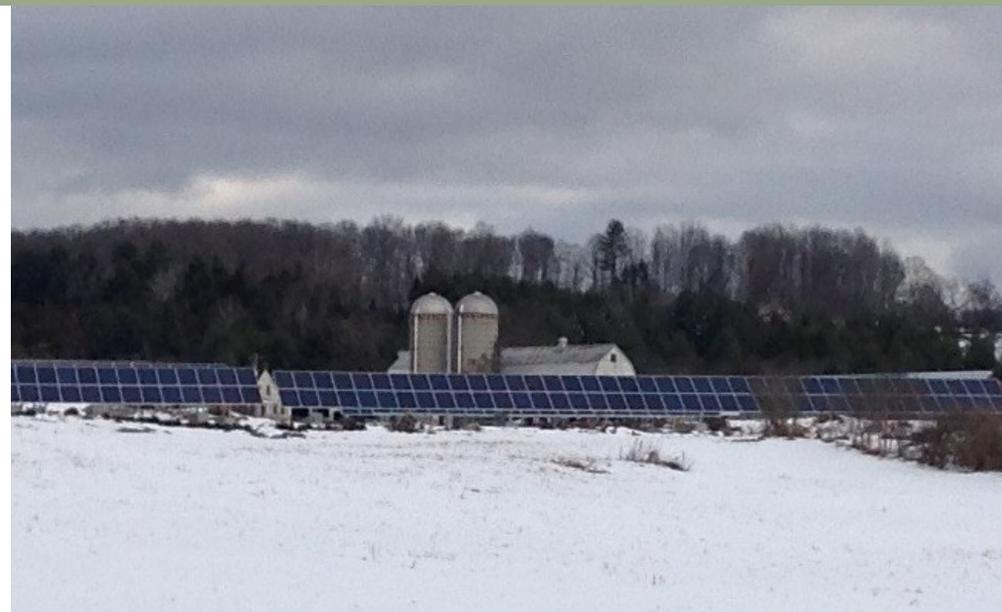
*McKnight Farm solar array in East Montpelier, showing about one quarter of the 1.5-acre array, which is rated at approximately 95 kilowatts power output. The system was built by Catamount Solar.*
