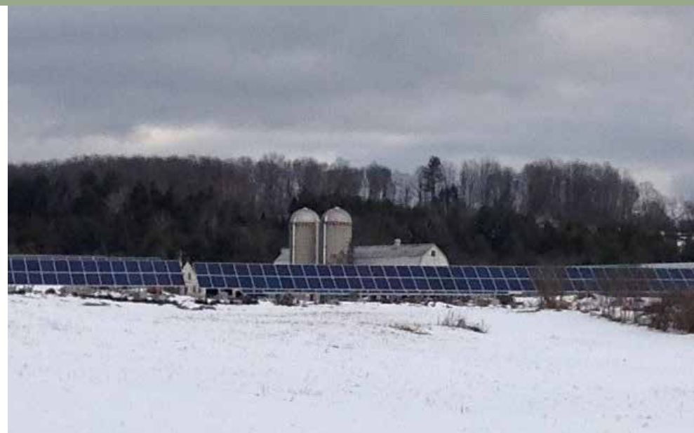
McKnight Farm solar array in East Montpelier, showing about one quarter of the 1.5-acre array, which is rated at approximately 95 kilowatts power output. The system was built by Catamount Solar.
