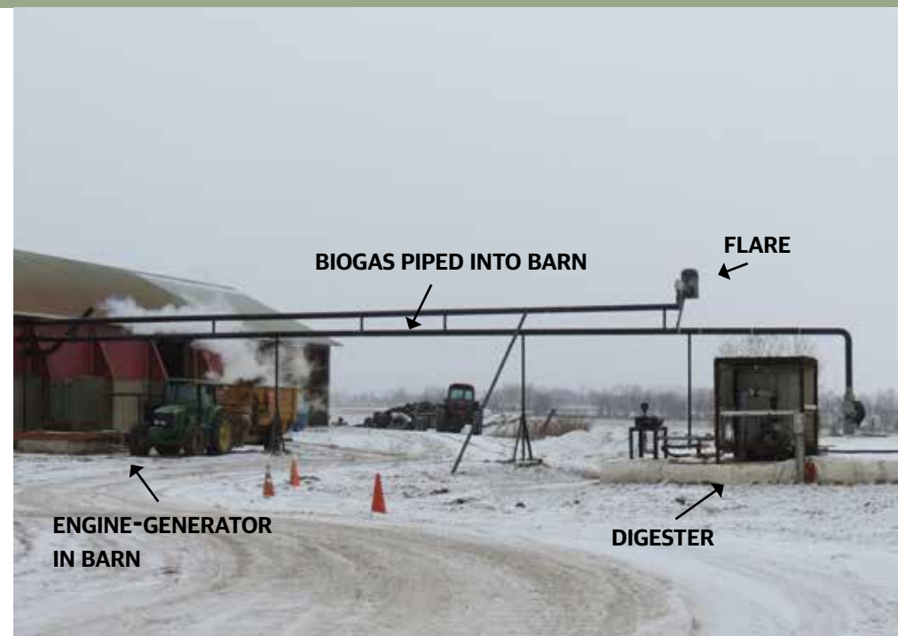
The engine-generator is housed in the building at the left. To right is the digester, part of which can be seen protruding above the ground. A pipe emerging from the digester carries biogas to the engine, and another pipe can be seen leading to the flare, used to burn the biogas in case the engine is not able to take the biogas.
