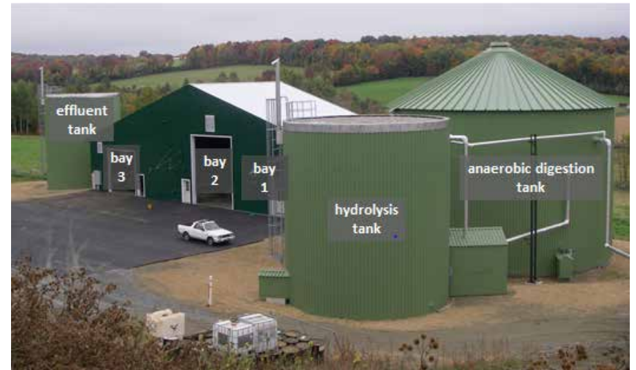
The Vermont Tech community anaerobic digester uses farm manure and food residuals to generate electricity, heat, and recycled nutrients.
