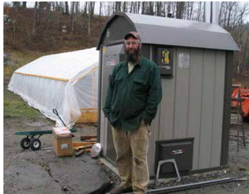
Paul Betz uses the Central Boiler eClassic to heat two greenhouses with cord wood.
