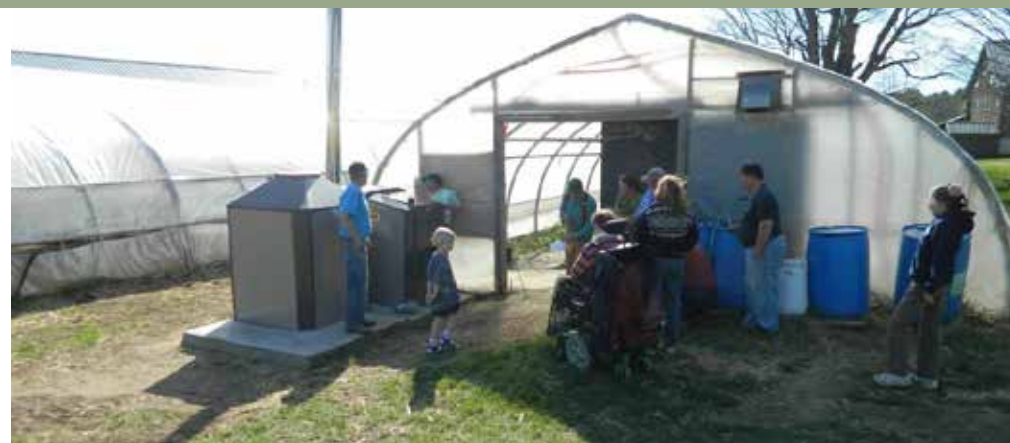
The Central Boiler Maxim 250 boiler installed at River Berry Farm in Fairfax, VT. These boilers may look like outdoor wood boilers common around Vermont, but they are EPA Phase II qualified due to improved emissions controls.
