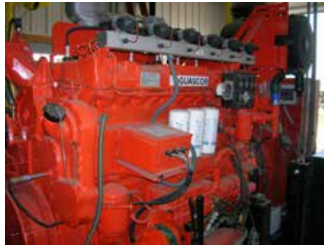
Guascor engines are commonly used with methane digesters in Vermont.
