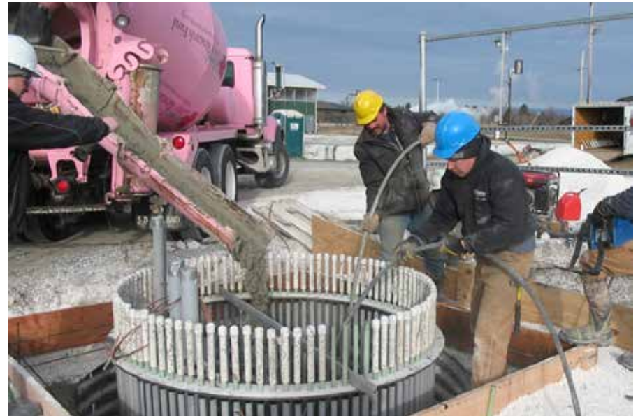
A below-ground pad of reinforced concrete is connected to a ring of rods (the "bolt cage"), visible in the photo, that rise to a few inches above ground level. This ring will also be encased in concrete, except for the top few inches, onto which the tower is bolted. Also shown are the electrical conduits, which will come up through the concrete floor inside the tower.
