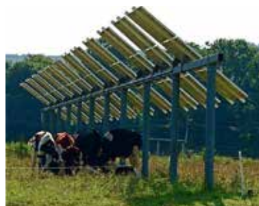
Steers on pasture underneath solar panels mounted on livestock-tough poles in South Deerfield, MA.
