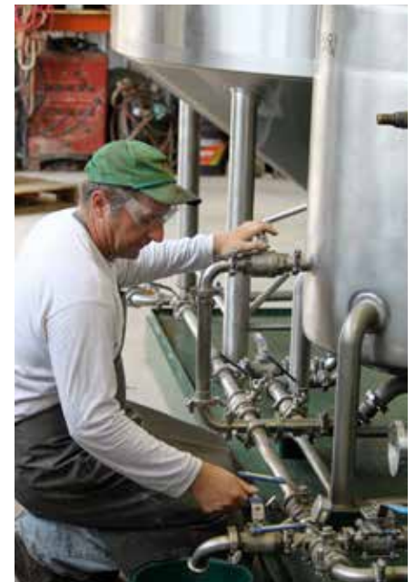
State Line Biofuels in Shaftsbury has been a pioneer in biodiesel development in Vermont.
