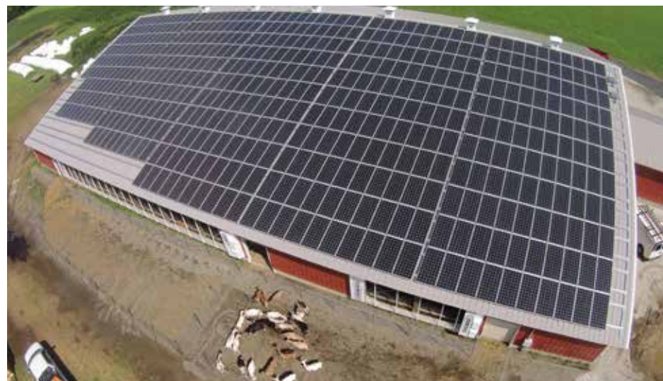
The 572 solar panels, here shown almost fully installed, use the one-third-acre south-facing roof, mounted on a frame designed by Aegis Renewable Energy.
