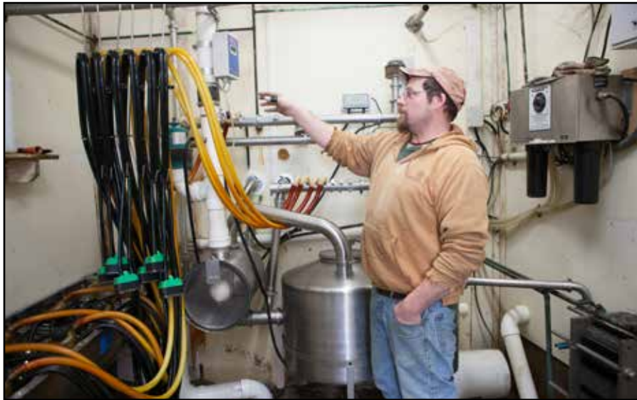
Alex explaining how the variable frequency holds the vacuum level on his milk pump.
