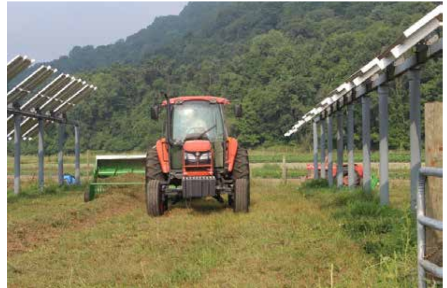
The dual land use pole and spline mounting system patented and installed by Hyperion Systems, LLC, Amherst, MA, demonstrates the possibility of baling hay between rows of solar panels on a farm in South Deerfield, MA.
